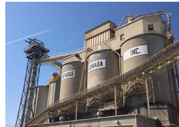
Lafarge Silos on Polson Quay
