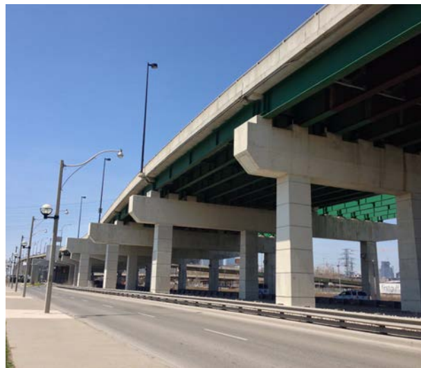
F. G. Gardiner Expressway and Lake Shore Boulevard East looking westward at Saulters Ave
