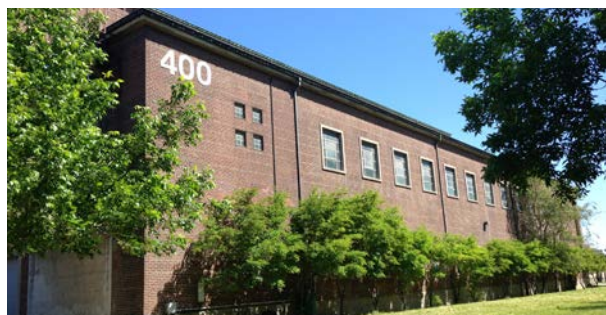
400 Commissioners Street Transfer Station
